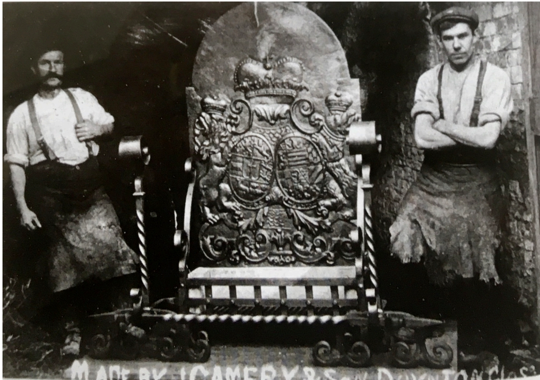
Fig 5.26. Joshua Camery, blacksmith and publican, was so proud of this work that he had postcards made. The fireback and basket were thought to be for Syston Court c 1905.
